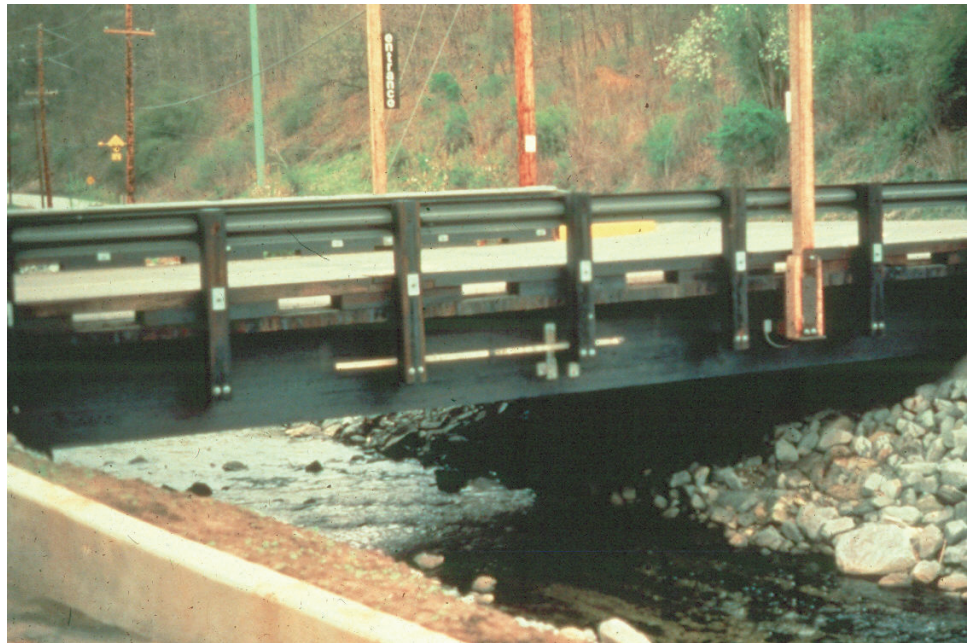
Figure 2.1.1 Glued-laminated Modern Timber Bridge
